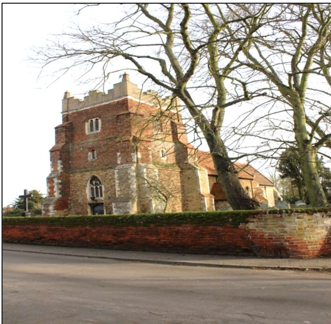
St Mary's Church, Tollesbury
